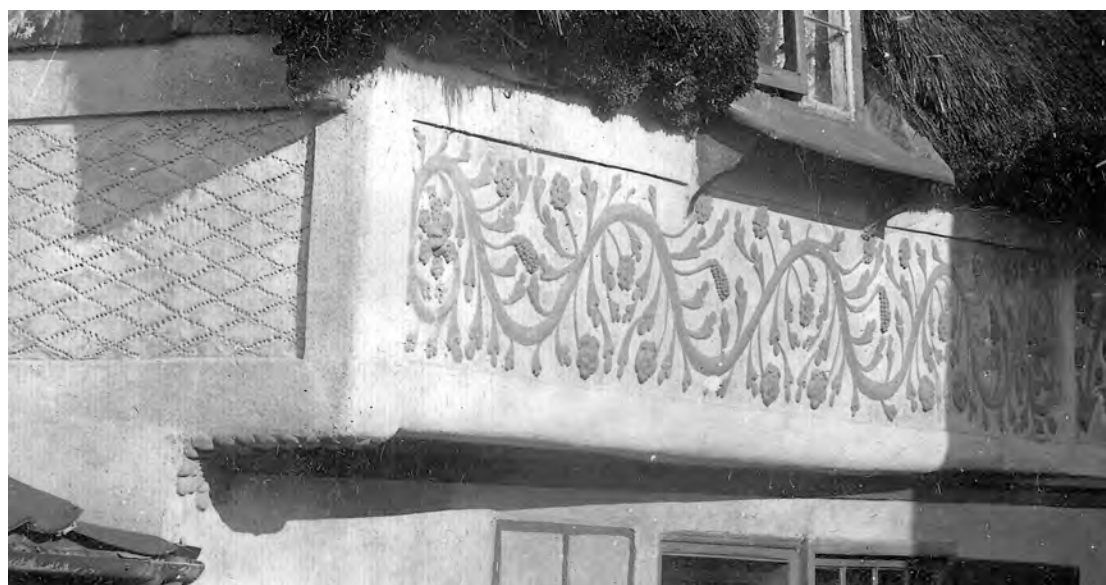
Fig 10. Photo of c1910-15 by Herbert Cave showing the decorative plasterwork painted in a single mid-tone, possibly the green mentioned in the 1949 article, see Fig 12.
