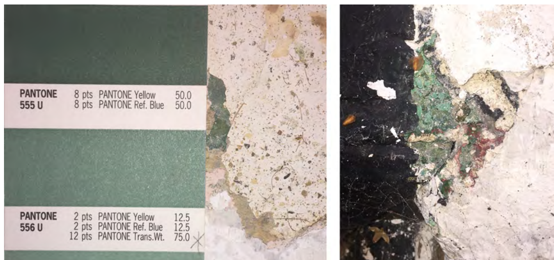
Fig 12. Remnants of this green pigment can be found along the full length of the decorative plasterwork, and under the layers of lime-wash from the early 1950s onward that covered over the area of the fresco band. It is possibly the single mid-tone colour paint shown in Fig 10 and described in the 1949 article. The black paint could have been painted over it to add contrast to certain areas.
