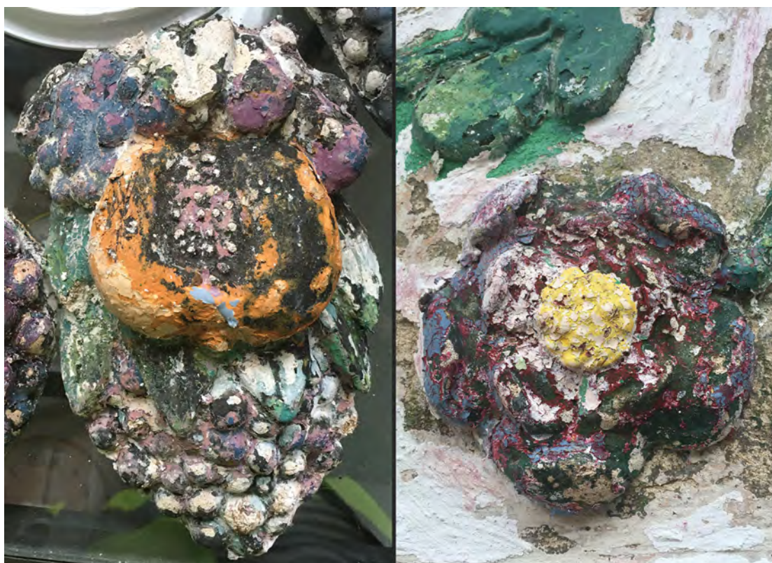
Fig 26 One of swag-tails (left) and one of the Tudor roses (right), the multiple layers of paint reflect the changing fashions and paint technology over the last 115 years.
