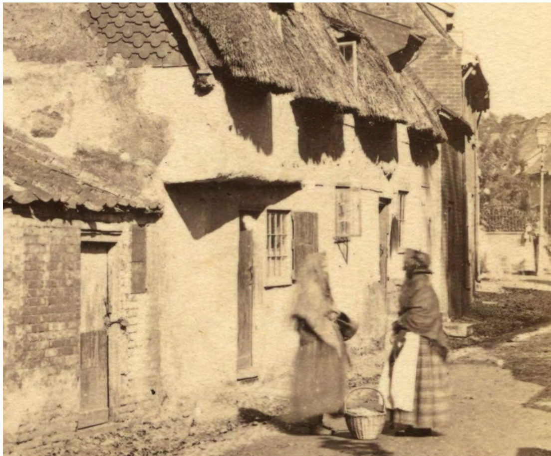
Fig 1. The first known image of the cottages is a photograph by W. Brunton, it is dated from the style of the women's clothes to between 1860 and 1875. There is no sign of painting on the front of the cottage only shadows cast by the form of the plasterwork.
