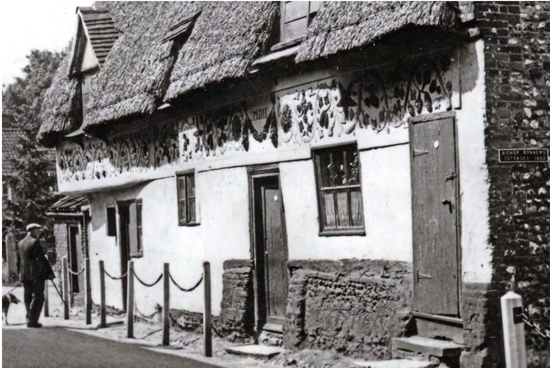
Fig 13. Cottages after 1949 but before re-thatch of cottages summer 1954
