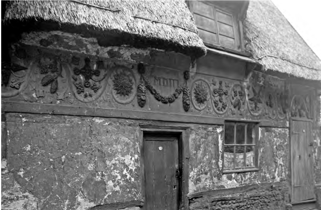
Fig 11. A photograph taken by George Plunkett in 1948 showing the green and black paint on the plasterwork with the fresco band just visible. This is the last photograph that faintly shows the fresco band, after this it was lime washed over.
