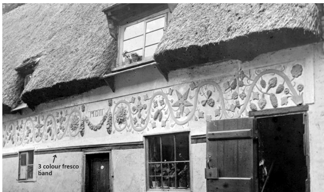
Fig 8. One of the photographs published in the article by Argent in 1906 showing paint on the pargeting for the first time.
